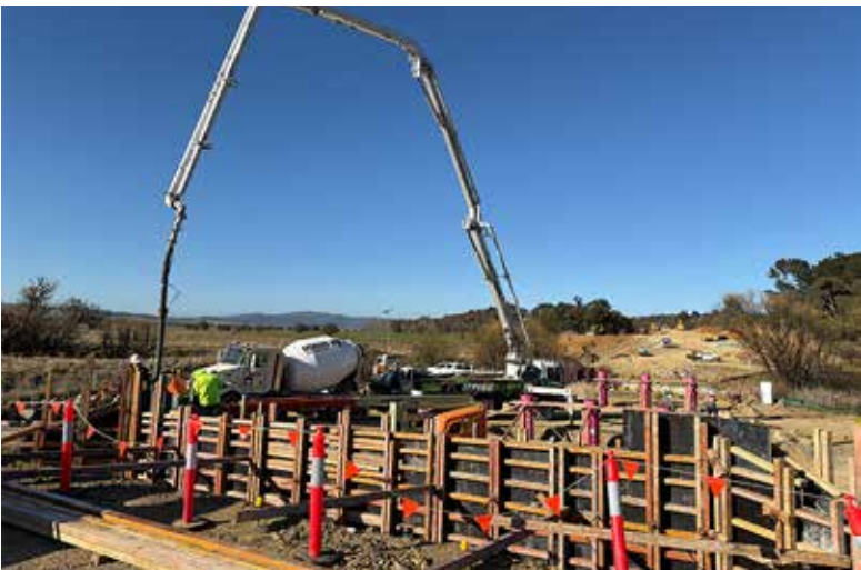
due to “frequent wet weather and unsuitable ground conditions.” Council received the grant funding from the NSW Government to upgrade Briars Sharrow crossing to a concrete bridge structure. The new bridge will be 92m long, 9m wide and will be constructed 4m higher than the existing crossing. Above: works continue. Photo QPRC
