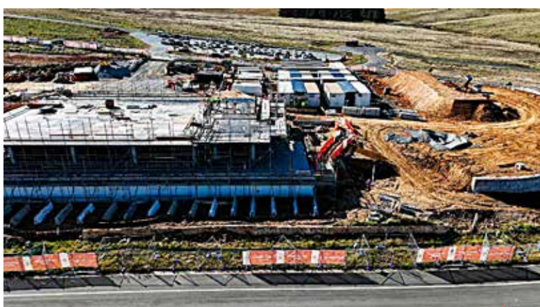
Phone: 1300 482 651 schoolinfrastructure.nsw.gov.au Above: construction is progressing on Block B. Image School Infrastructure
